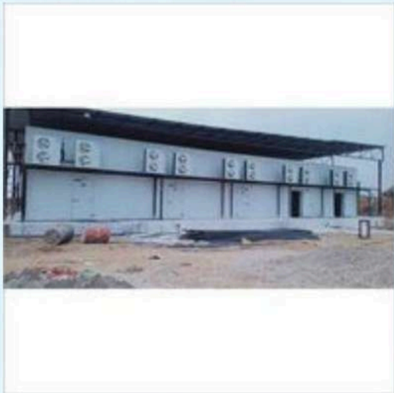
Mushroom Cold Storage Plant
