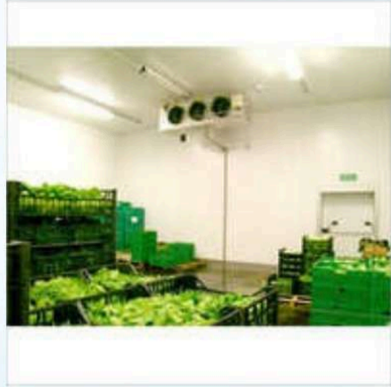
Vegetables Cold Storage Room
